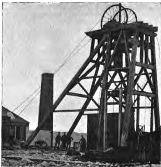
FIG. 531.—Wood pit-frame.
